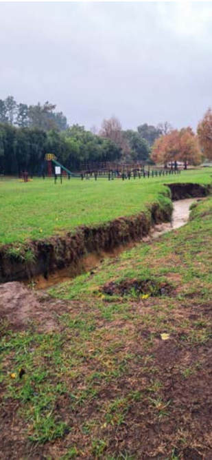
Sloot to get a shake-up: The City has shared its plans to upgrade the Geelsloot ponds in Somerset West with the public. The project will ultimately curb flooding downstream.
